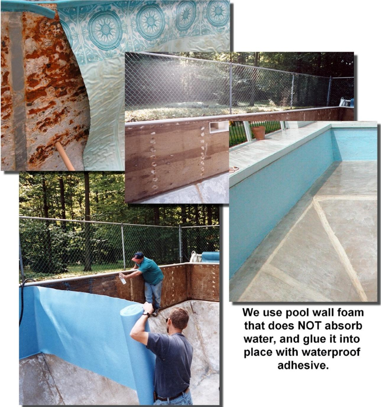
**We use pool wall foam that does NOT absorb water, and glue it into place with waterproof adhesive.**
