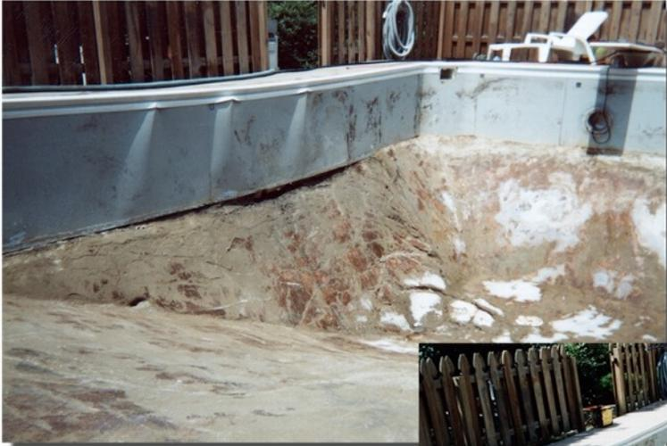
This bottom has ground water damage but is fully repairable. All loose pieces and soft areas will be removed and a cement/vermiculite pool bottom mix will be troweled into place.
