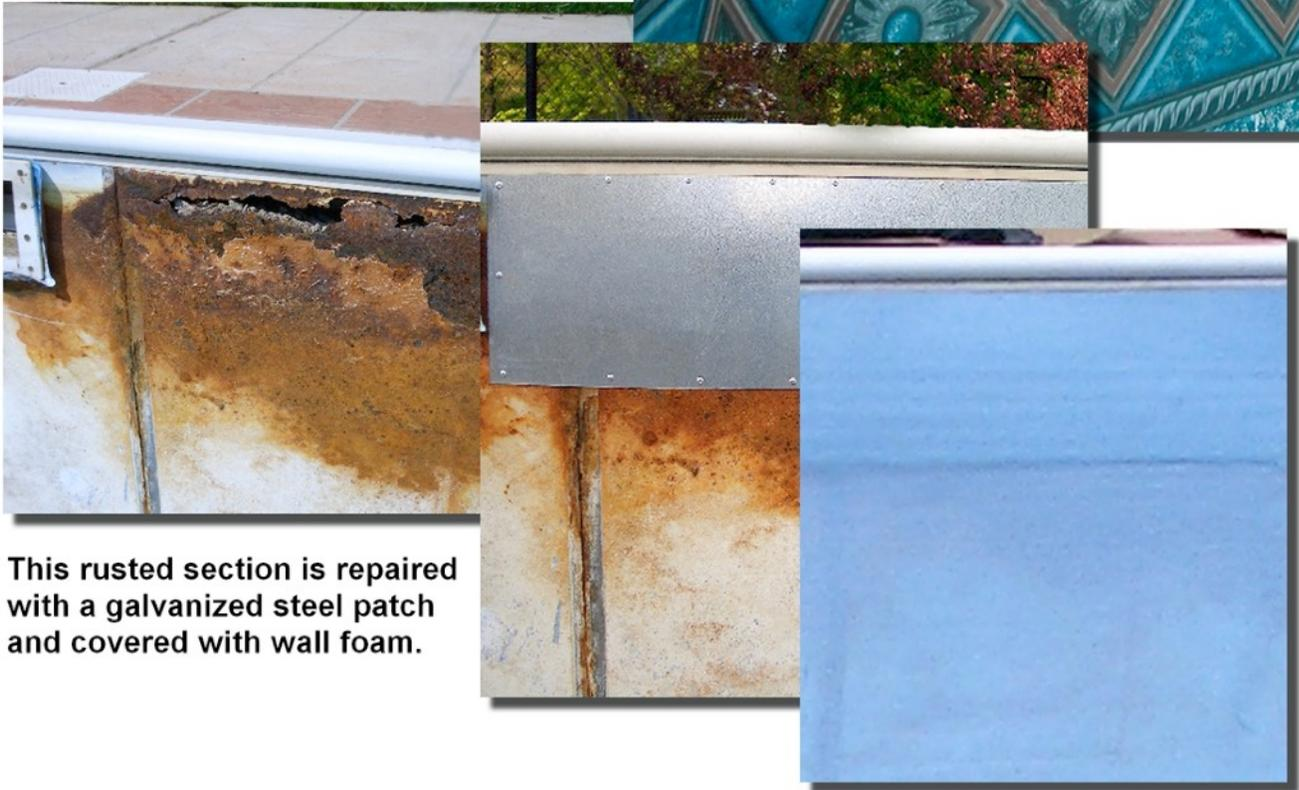
This rusted section is repaired with a galvanized steel patch and covered with wall foam.
