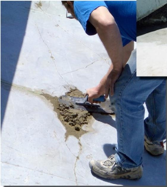
This pool's bottom was extremely thin in some areas, and required spot patching with sand and cement.
