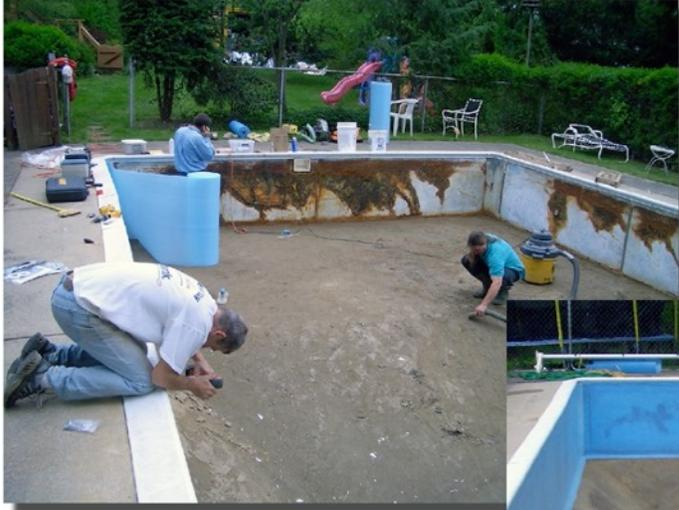
This sand bottom was carefully cleaned by hand, and then trowled smooth just before the liner was fitted.
