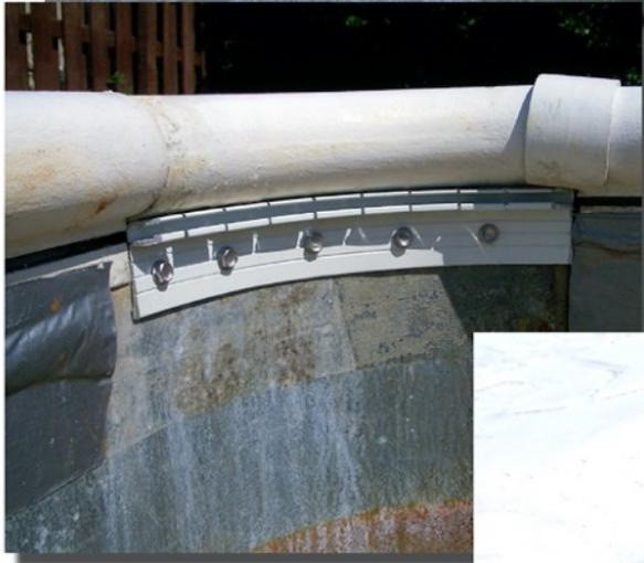
A new piece of aluminum corner tracking is installed with stainless steel fasteners.
