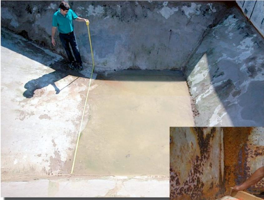
Photos, such as these, are sent to the factory; enabling them to make a better fitting liner.
