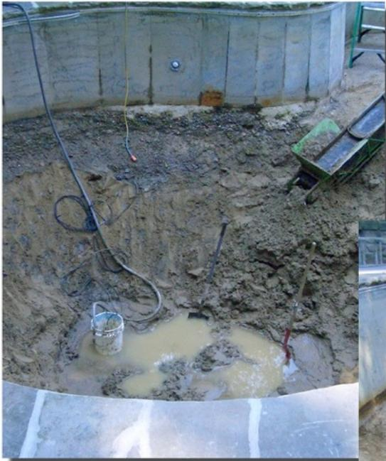
This pool's bottom was reshaped, and a new hard bottom installed.
